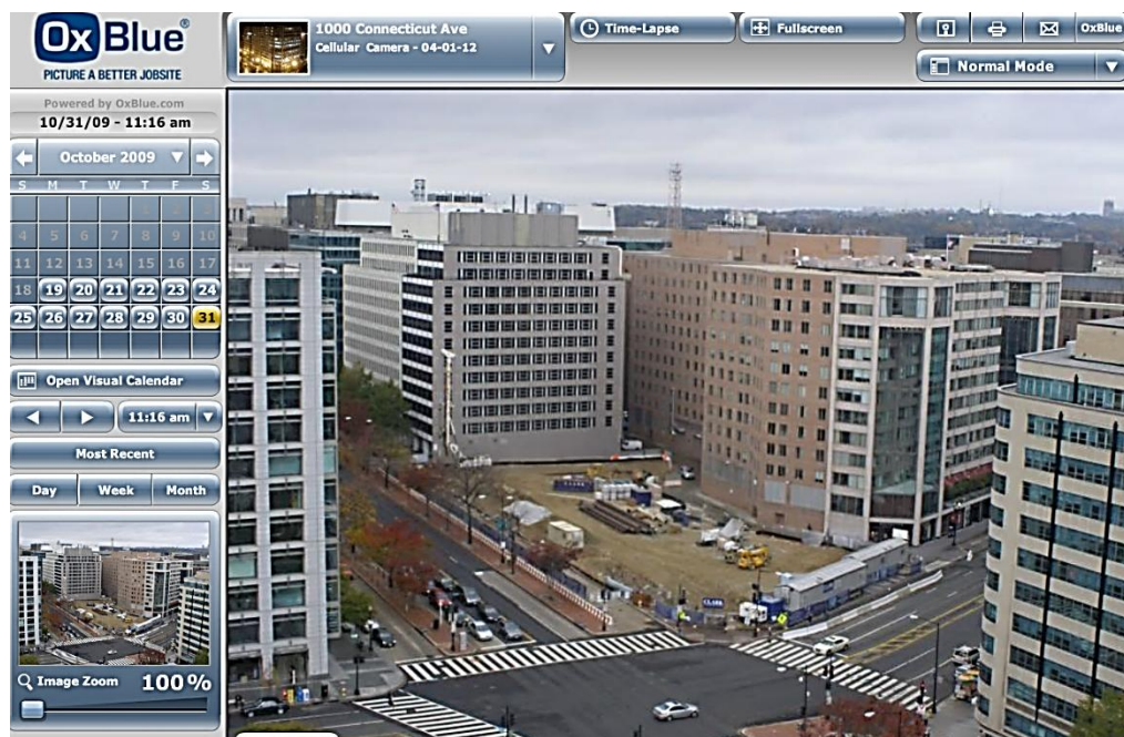
Figure 56 construction site before excavation (October 2009)
